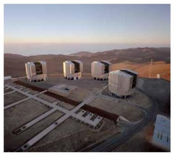
8.2 m four telescopes of the Very Large Telescope of ESO (European Southern Observatory), usable as an interferometer (VLTI). Cerro Paranal (Chile)
